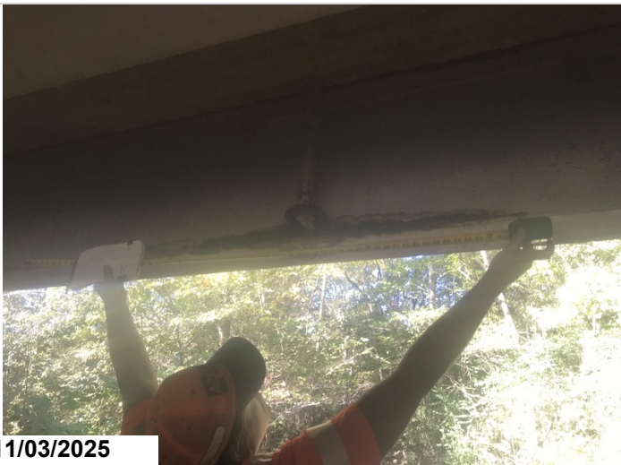
Girder 1, Adjacent to abutment 2, Under scupper: 5' area of corrosion with flaking rust and up to 1/8" section loss. 5LF CS3
