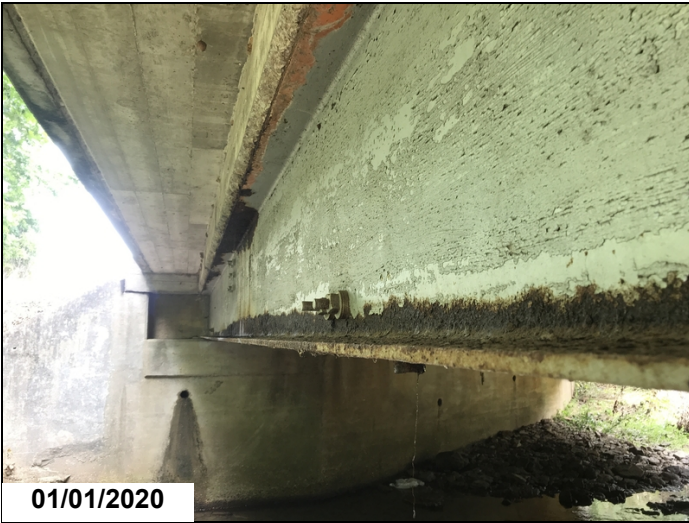
Beam # 1 with active corrosion and initial section loss.
