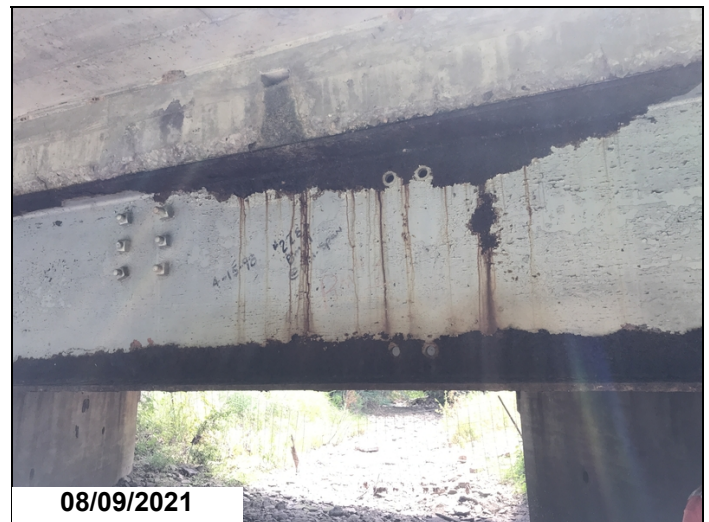
Beam # 1. Corrosion.
