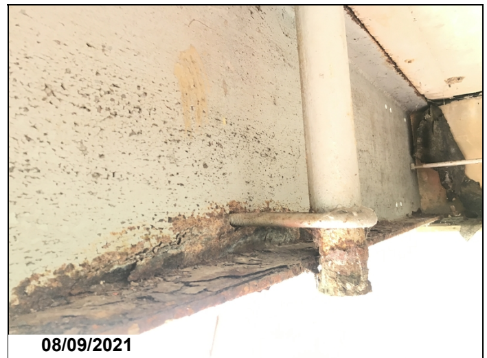
Beam # 14 corrosion.
