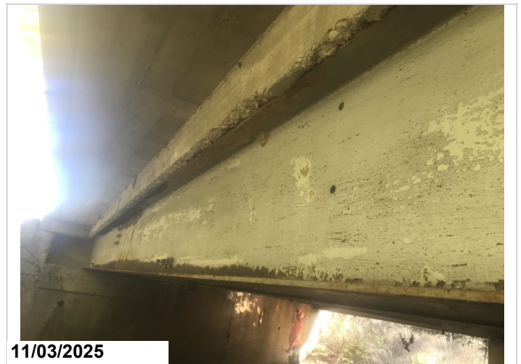
Left edge of deck, Over exterior girder: Shallow spalling. 25SF CS3
