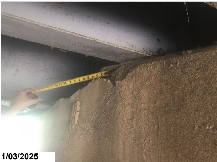
Abutment 2, Girder 3 bearing: Approximately 2" of bearing area loss. 1EA CS2
