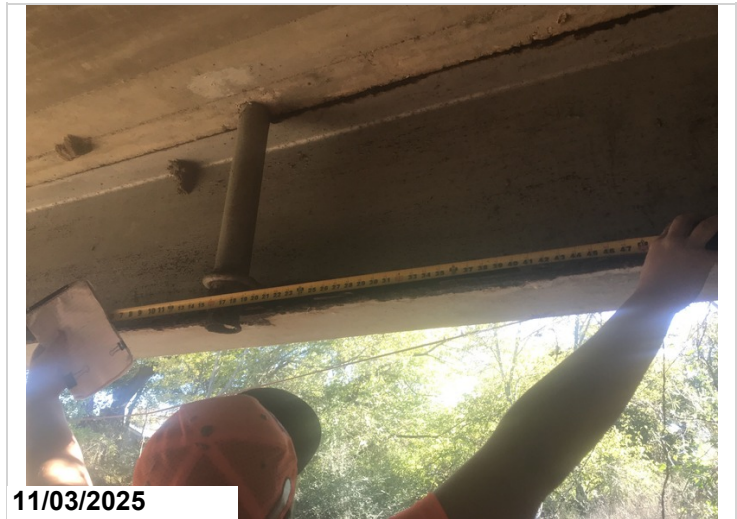
Girder 14, Adjacent to abutment 1, Under scupper: 4' area of corrosion with flaking rust and up to 1/8" section loss. 4LF CS3
