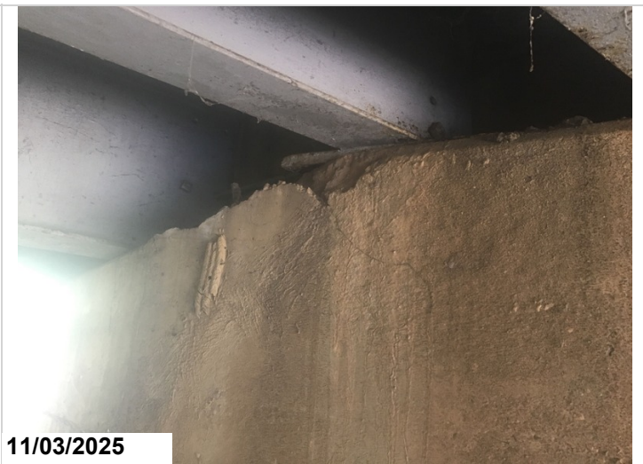
Abutment 2, Under girder 3 bearing: Concrete deterioration/spalling with approximately 2" of bearing area loss & exposed reinforcing steel. 1LF CS3 spall
