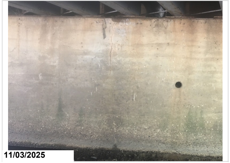
Abutment 2, Centerline: Vertical crack. 1LF CS3
