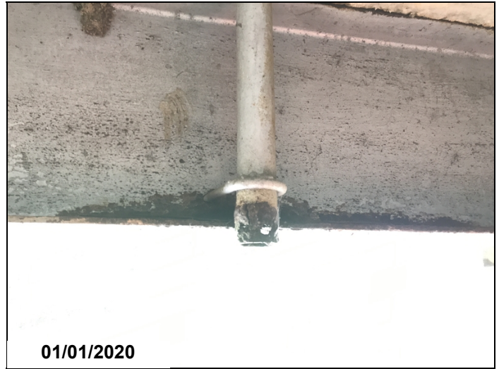
Beam # 14 adjacent to Bent # 2 has active corrosion with initial section loss.
