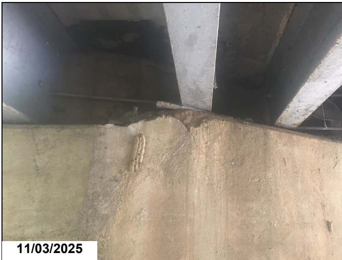
Abutment 2, Under girder 3 bearing: Concrete deterioration/ spalling with approximately 2" of bearing area loss.
