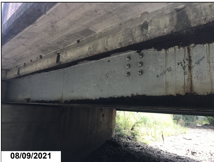
Beam # 1 corrosion.
