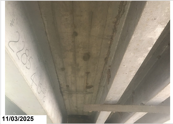
Deck undersurface, Bay 2: Transverse cracks with light efflorescence. 4SF CS2
