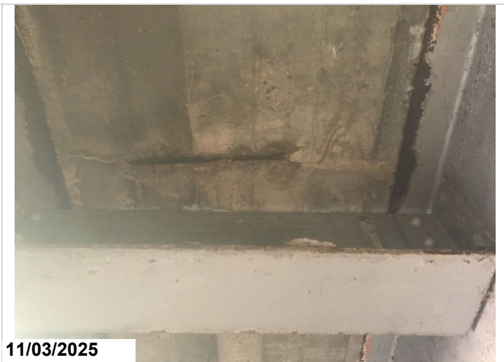
Deck undersurface, Bay 1, Adjacent to diaphragm: 14" spall with exposed reinforcing steel. 2LF CS3
