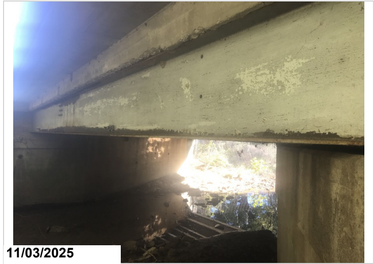
Girder 1, Exterior face: Approximately 20' long area of active corrosion with flaking rust. 20LF CS3
