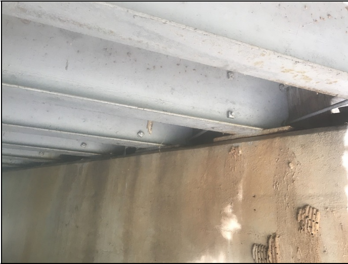
Abutment 2, girder ends and bearings.
